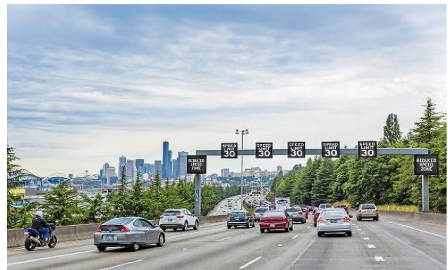
Design of an optimal variable speed limit control system for relieving congestion at bottlenecks
