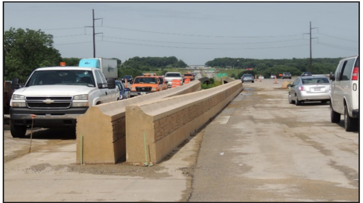
Figure 4. Implementation of the new concrete median barrier in Iowa. Note that the top of the barrier is more tapered than traditional designs. This new design reduces the probability of a vehicle occupant's head making contact with the barrier in the event of a crash.
