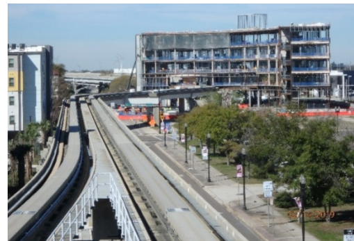
View of existing elevated guideway
