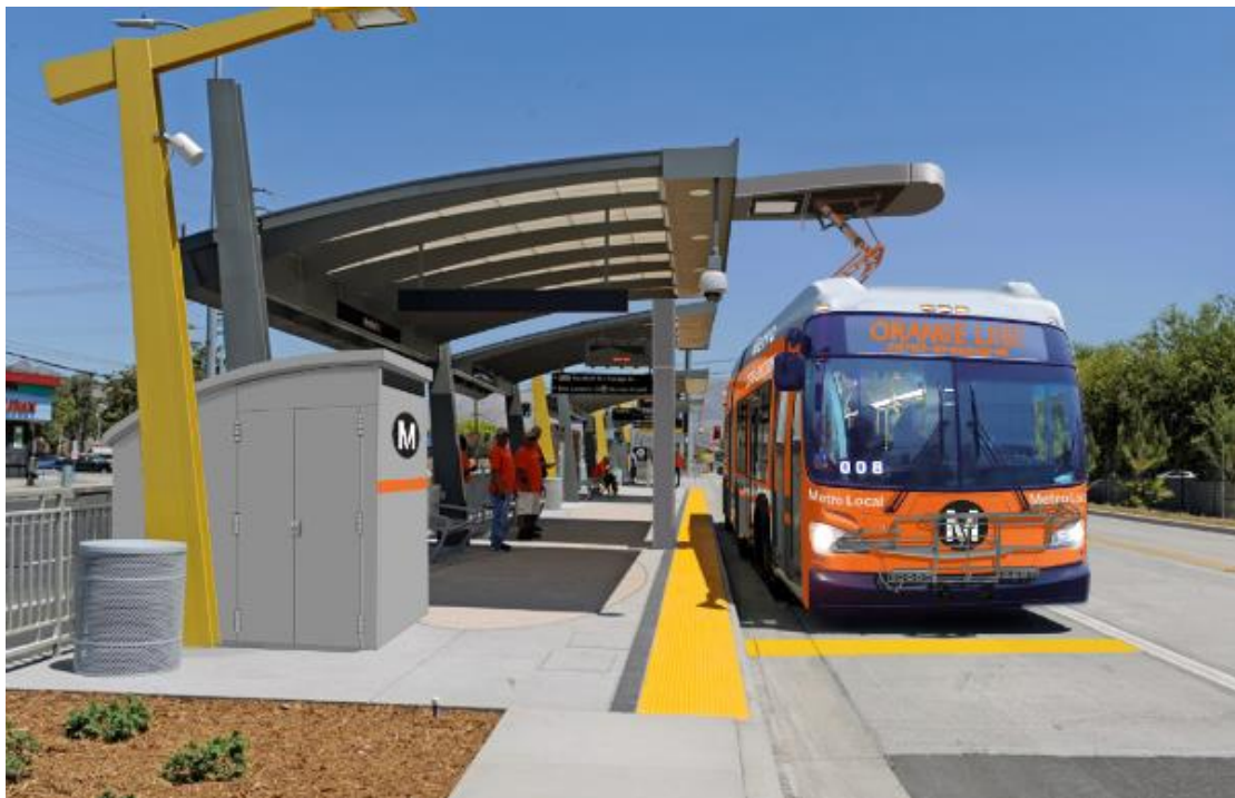
Figure 1. Orange Line Electric Bus with SAE3105-1 Charging Station
