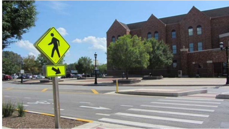
Figure 4. Complete streets improvements were made in 2013 on Main Street in Urbana, IL. The improvements included this pedestrian crossing, with a refuge island. Image courtesy of Champaign County Regional Planning Commission. (Source: FHWA Case Studies in Delivering Safe, Comfortable and
