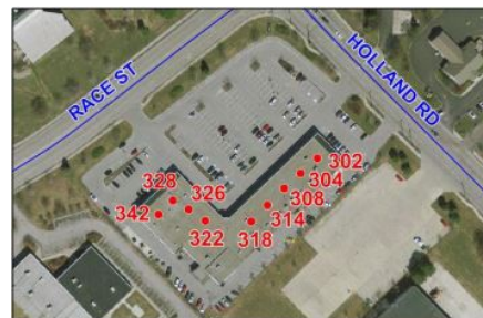
Structure - Interior Unit Location
