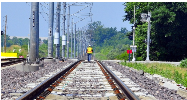
Figure 1: Manual inspection of railway tracks
