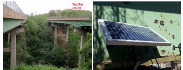
Figure 4: I-95 Bridge site and the solar-wind hybrid power
