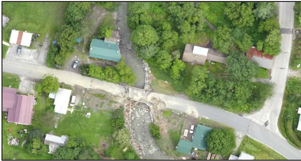
Figure 4: Woody debris damage to one of the bridges in Plainfield, VT caused by severe storms that hit the area in July 2015
