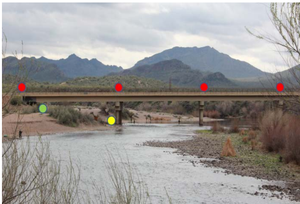
Figure 1: Local bridge structure
