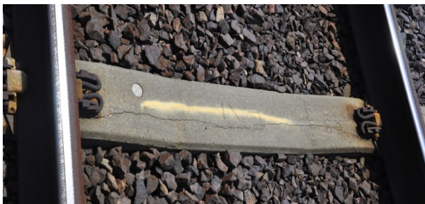
Figure 2: Concrete ties, fastening systems and ballast
