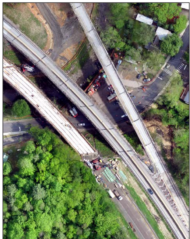
Figure 3: UAS mapping of an active construction site
