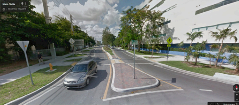
Before and after view of a Complete Streets project on 27th Street.
