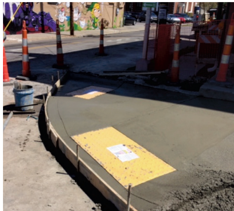
Pedestrian Safety Improvement under construction at 6th Street and North Limestone in Downtown Lexington, KY.
