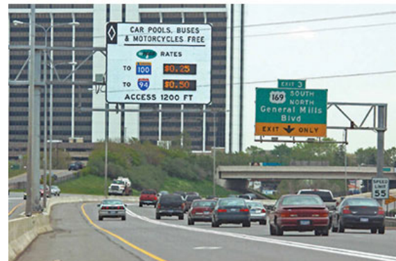
Figure 1: In Minneapolis, MN, a variable message sign above the I-394 HOT lanes shows current toll rates Source: FHWA and MnDOT
