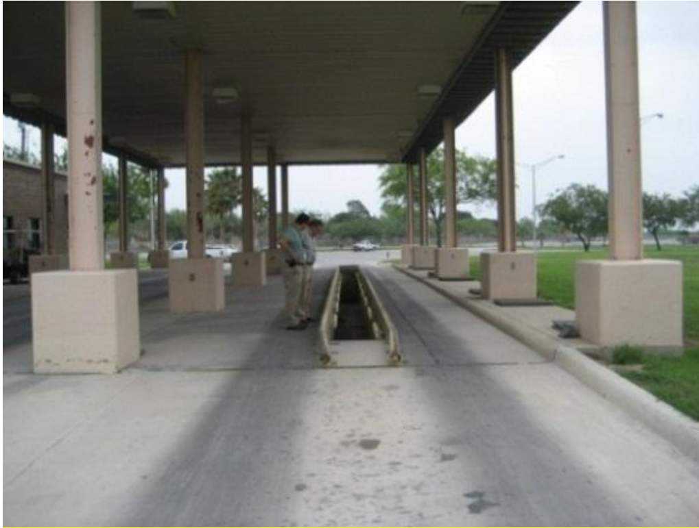
Above: Rio Grande City, TX. This inspection pit is typical for what is planned for each border facility inspection lane.
