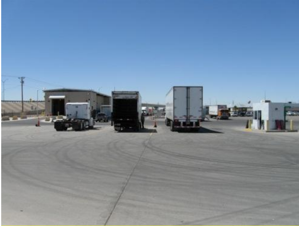
Above: Example of an exposed inspection area with no canopy or inspection pits.
