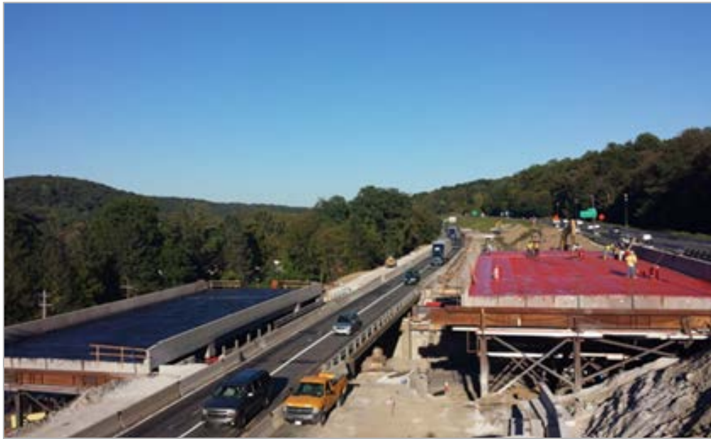
Figure 1 Dingle Ridge Road bridge replacement project using slide-in bridge construction method (New York State), Photo by FHWA
