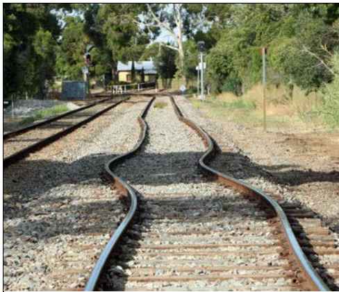
Figure 12 Buckling of a CWR.
