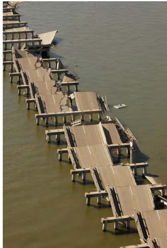
Hurricane Damage from Wave Action to Highway 90 in Bay St Louis, MS (Illinoisphoto.com)
