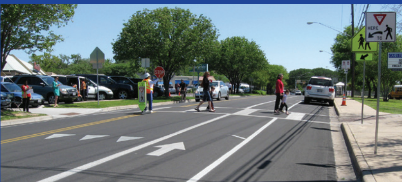
Newly constructed crosswalk.
