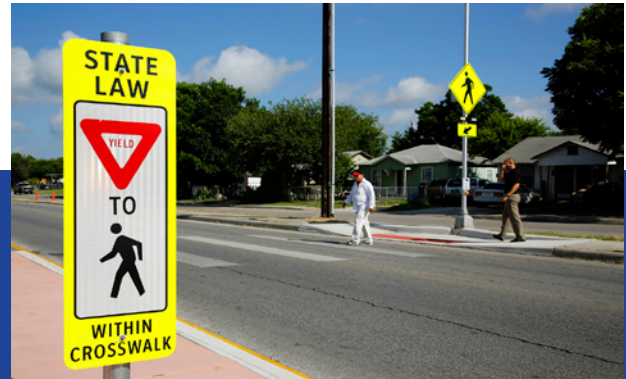
The newly installed Z-crossings and signage in San Antonio, TX, increase visibility of pedestrians to cars, making crossings safer.
