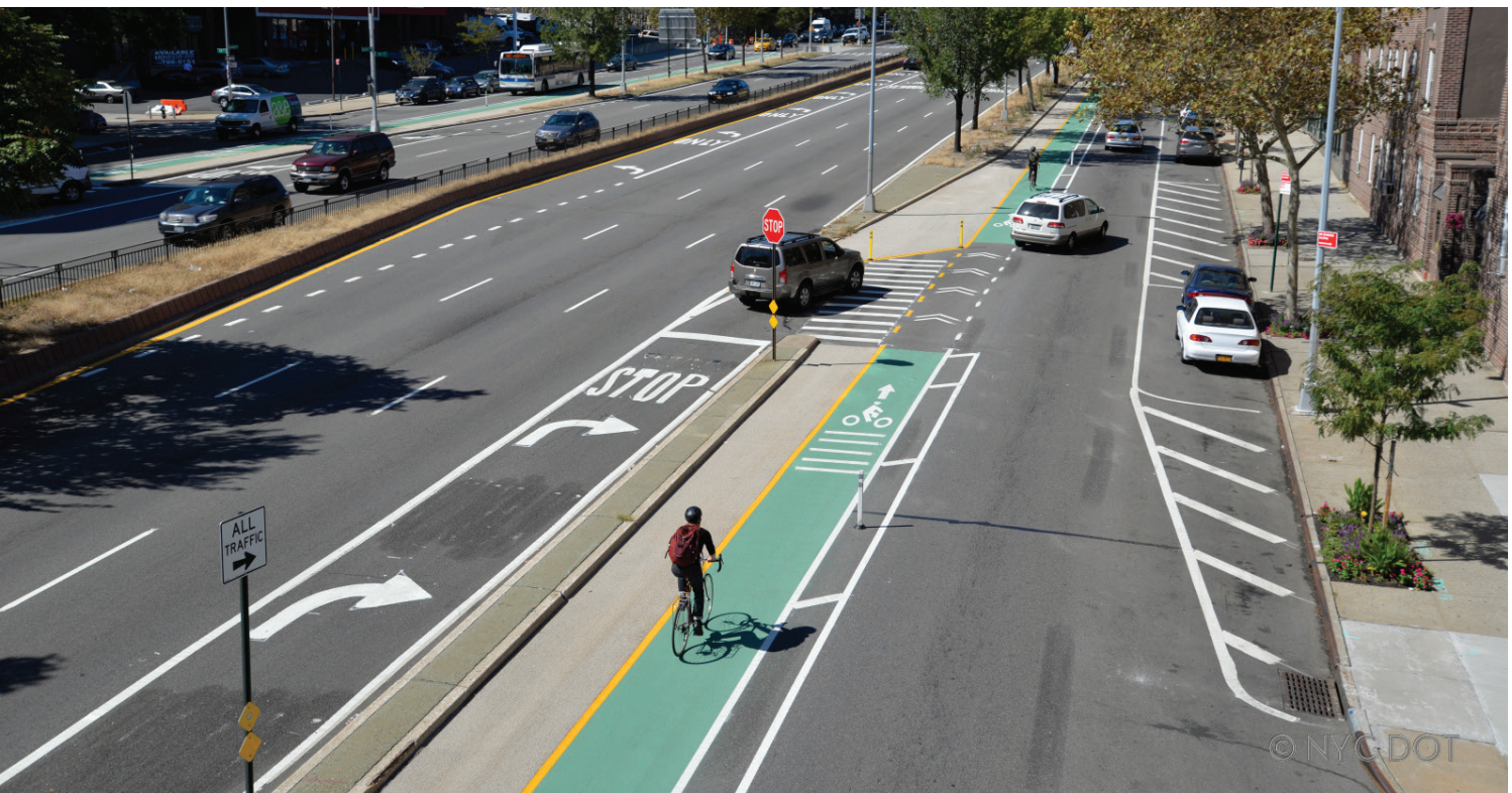
Model Complete Streets project on Queens Boulevard in New York City, requiring vehicles to stop, and not just yield, before merging across the pedestrian crossing and separated bike lane.
