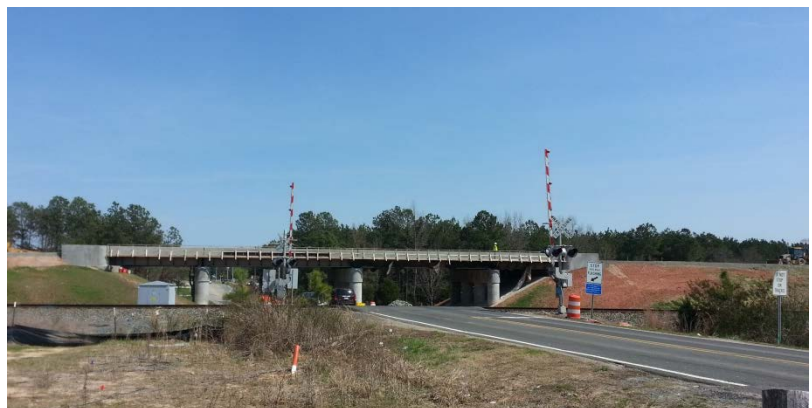
Grade Separation at Hopson Road in Morrisville, NC
