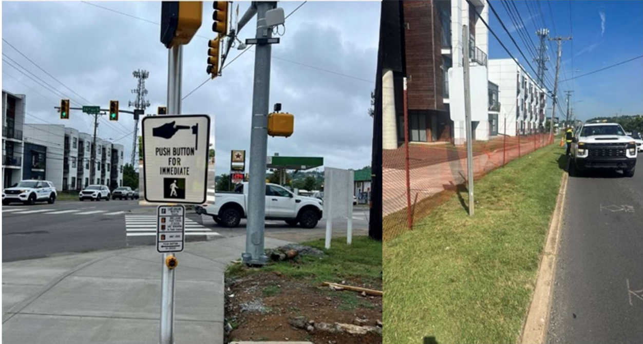
Figure 35 Temporary interventions were deployed on Clarksville Ave and 26th Ave. Left. The signal was modified to immediately prioritize pedestrians in response to ped calls. Right a temporary fence was installed to reduce out of crosswalk events at a problematic area.
