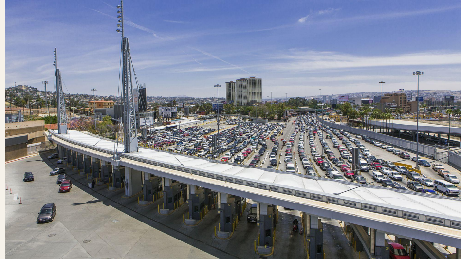
San Ysidro Land Port of Entry, California
