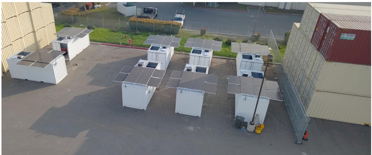
Figure 1- 8 Gen 2 Dock Systems under construction at CONEX West for the Phase 2 SOAR project.
