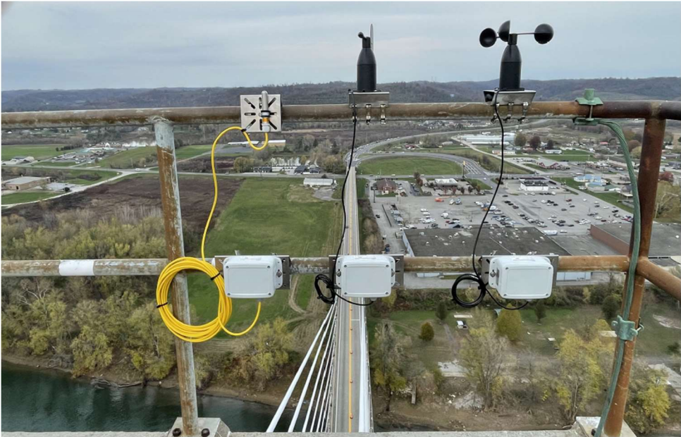
Figure 6 - Weather Station Installed at Top of the Bridge Tower
