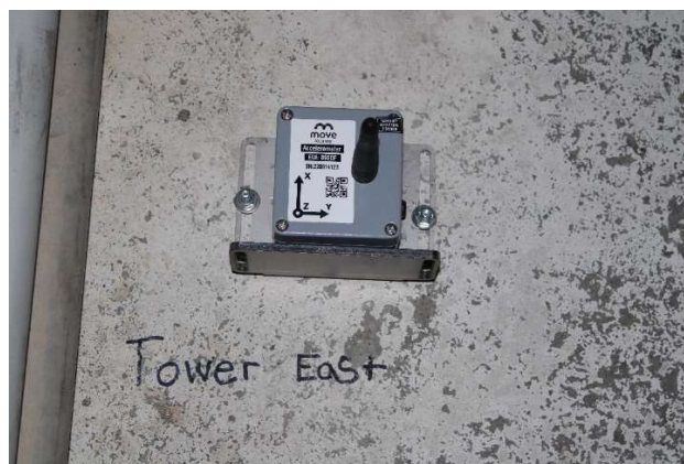
Figure 4 – Accelerometer Installed on Bridge Tower
