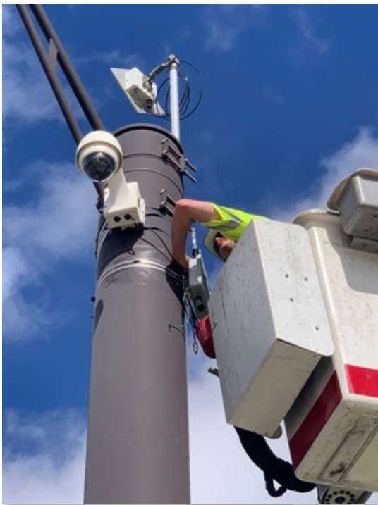
Figure 6. City of College Station Installing Equipment
