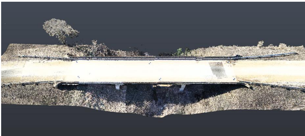
Figure 9. Point cloud data collected by Skydio drone in Saline County, Kansas
