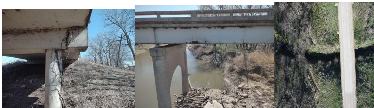
Figure 4. Sample bridges selected for full-scale implementation field test in Spring 2025
