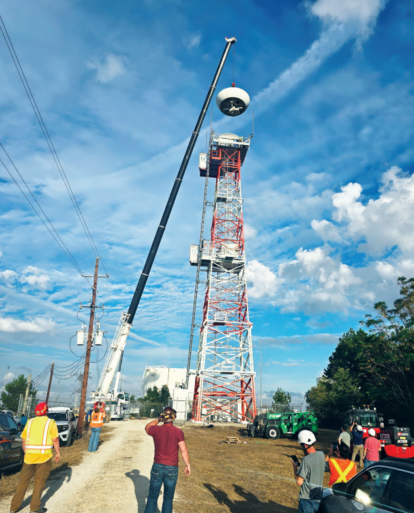
Surface Movement Radar installation at Houston Hobby International Airport
