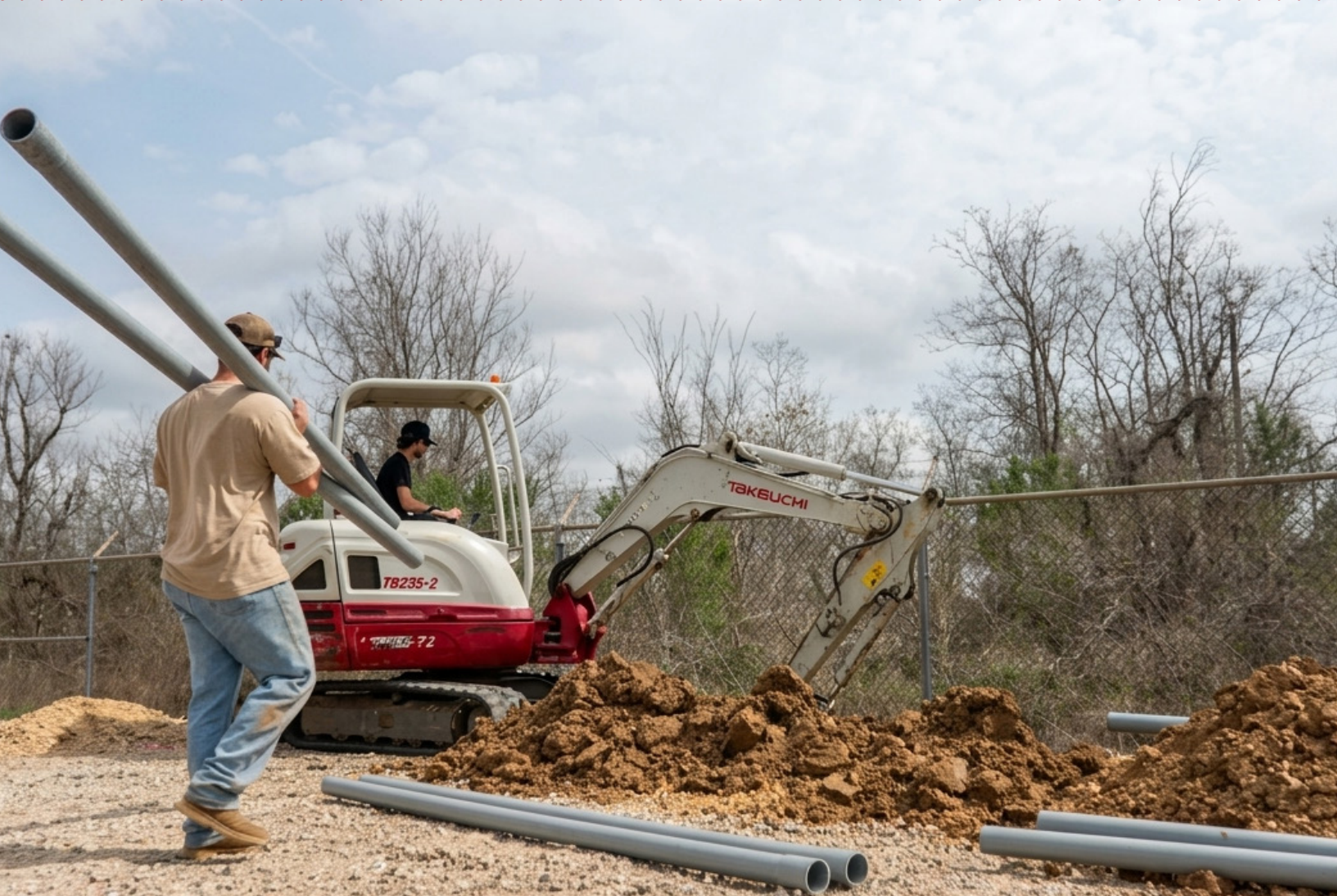
Telecommunications Infrastructure Replacement (TIR) at Houston Hobby International Airport
