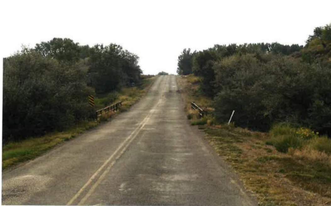
Figure 1 Antelope Creek Bridge
