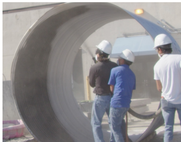
Figure 4. Work to extend the application of sprayable UHPC to Repair/Upgrade capacity of existing deficient steel culverts
