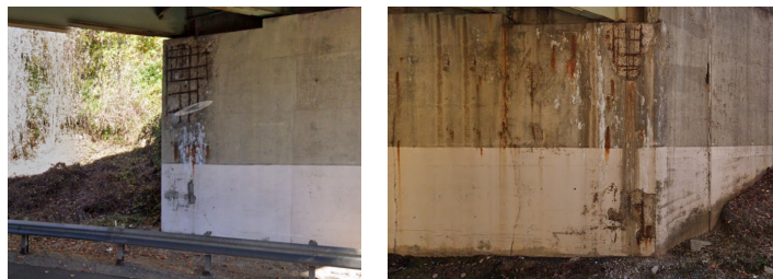
Figure 1. Two abutments partially repaired using Sprayable UHPC.
