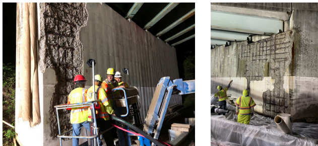
Figure 2. Condition of both abutments ready for spray process.
