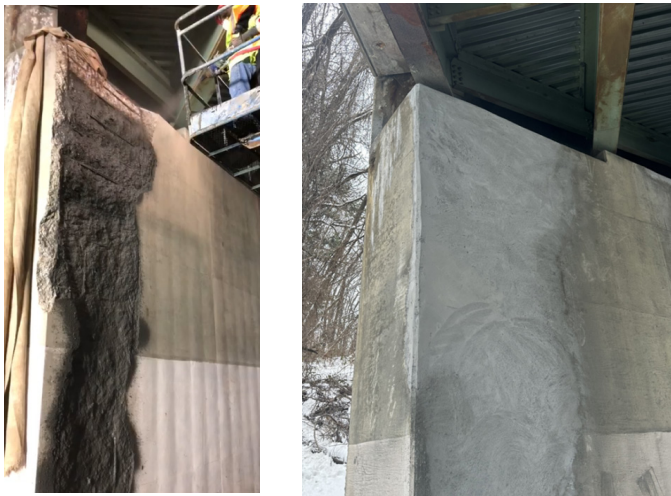
Figure 3. One of the abutments repaired using sprayable UHPC during spray process and the same abutment about four months after spray.
