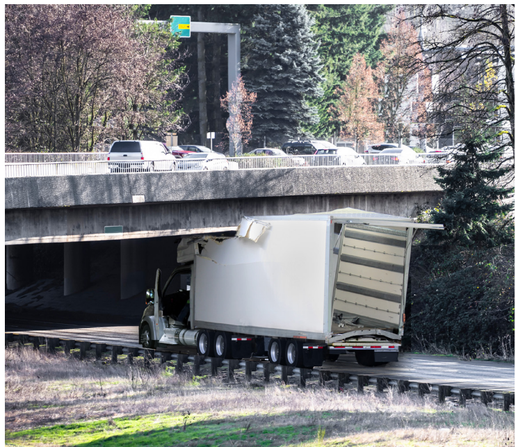
Figure 5: Damage caused by a truck driver overestimating the height of the overpass (courtesy of U.S. DOT)
