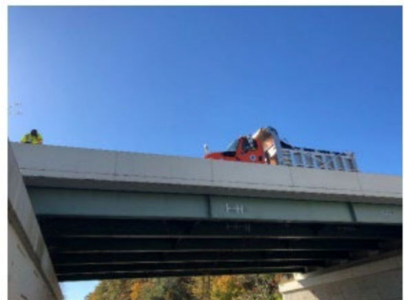
Figure 32. Loaded truck crossing a bridge during a load test. Source: CIAMATIS
