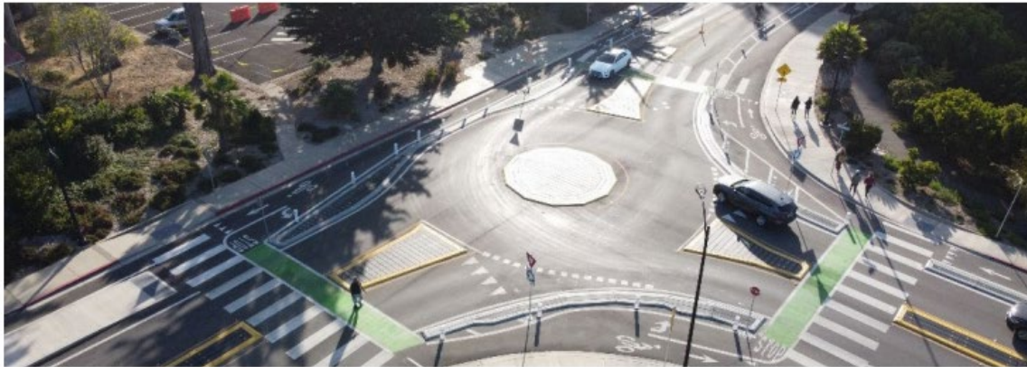
Figure 9. Mini-roundabout. Source: ZKxKZ, LLC
