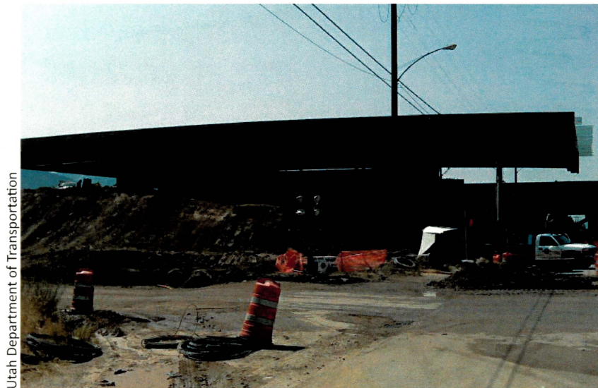
Bridge span nearing its final position
