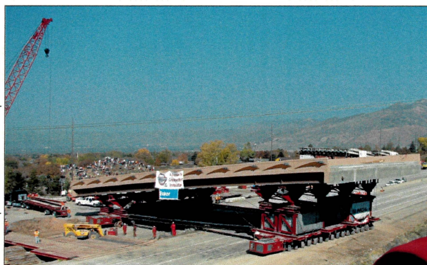
Bridge span being moved into place using a Self-Propelled Modular Transport (SPMT)
