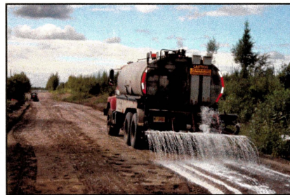
Applying chemical soil stabilizer to Horseshoe Lake Road.
