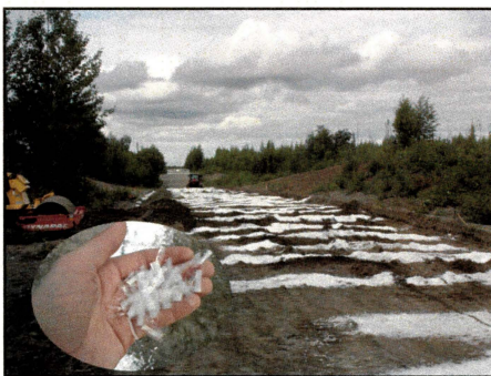
Applying geofibers to Horseshoe Lake Road near Wasilla, Alaska.
