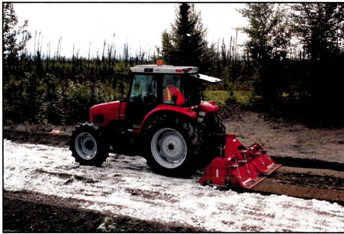
Mixing the fibers into the roadway on Horseshoe Lake Road.
