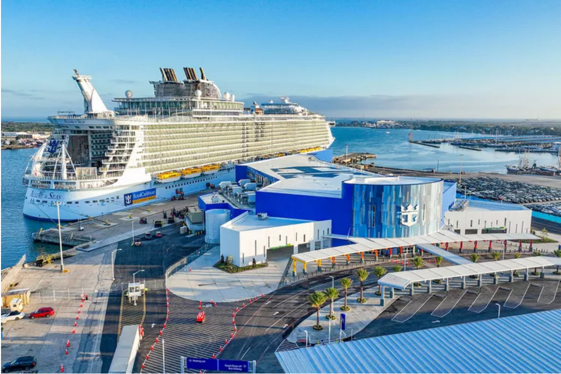
Figure 38: New Royal Caribbean Port of Galveston Facility 391
