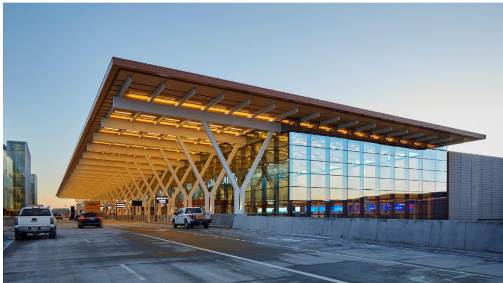
Figure 34: The New MCI Terminal 363
