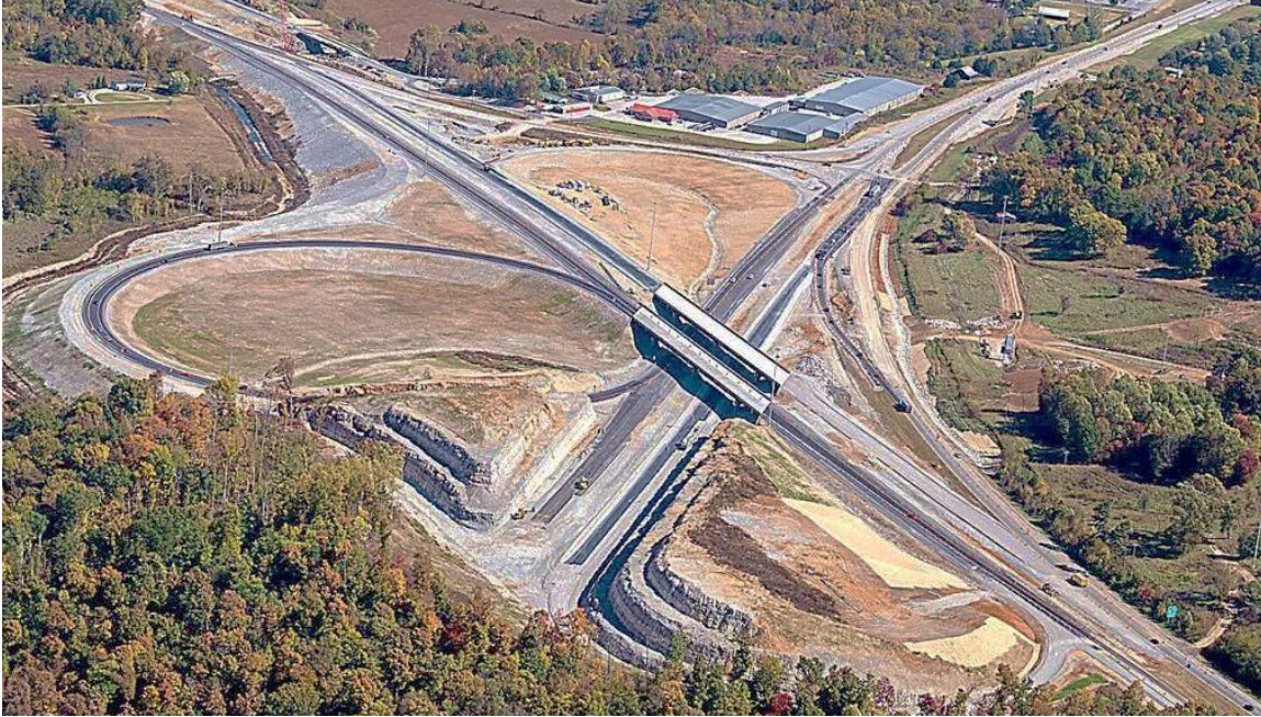
Figure 31: Interchange Work in Progress 345
