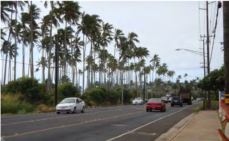
Figure 3-2. Kuhio Highway in East Kauai
