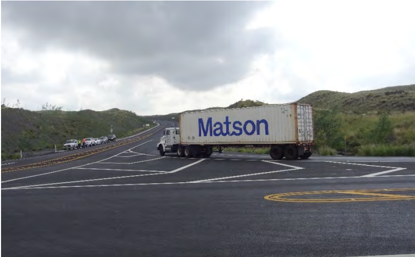
Figure 7-4. Container Truck Heading East on the Daniel K. Inouye Highway on the Big Island
