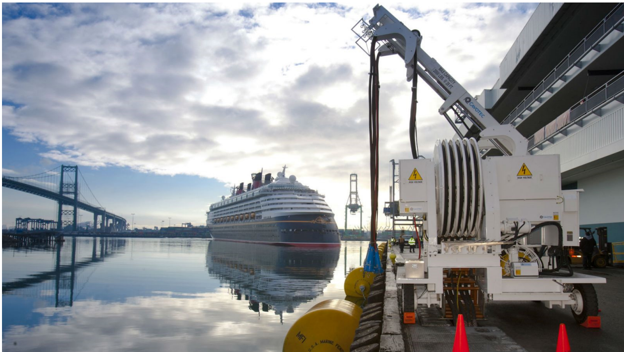
Electric shore power at the Port of Los Angeles (Image source: Maritime Executive)
