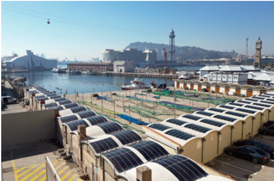
Solar film installed on rooftops in Barcelona (Image source: Optics.org)
