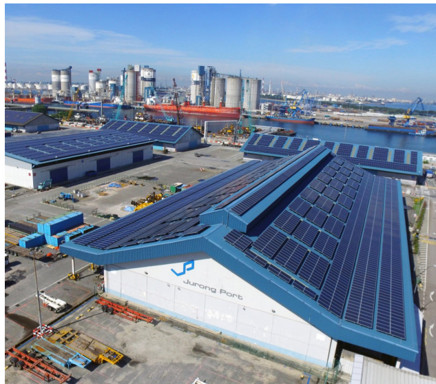
Solar panels at the Jurong Port, Singapore. (Image source: Maritime and Port Authority of Singapore)
