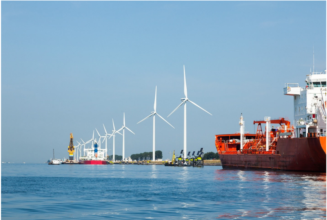
Wind turbines on shore at a port. (Image source: Adobe Stock)
