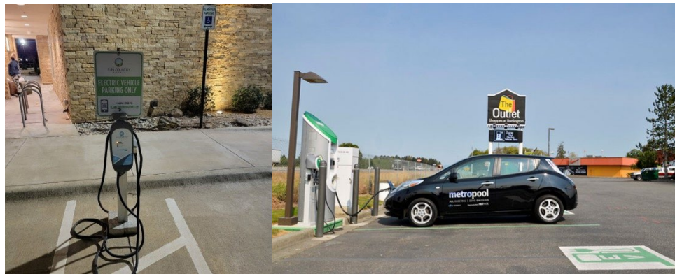
Figure 2-1: Level 2 chargers (left) are common in home, workplace, and public settings and can charge a BEV from empty in 4–10 hours. DCFC chargers (right) are common as public chargers and along highway corridors and can charge a BEV to 80 percent in under an hour. (Source: 123RF [left]; Washington State Dept of Transportation [right])
