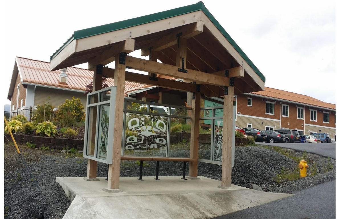
Saxman, Alaska, Senior Center bus stop. Source: FHWA
