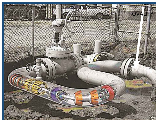
Smart Pig in use inside of a Pipeline
