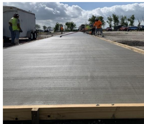
Construction of the Full-Scale, Jointless UTW-ECC Overlay
