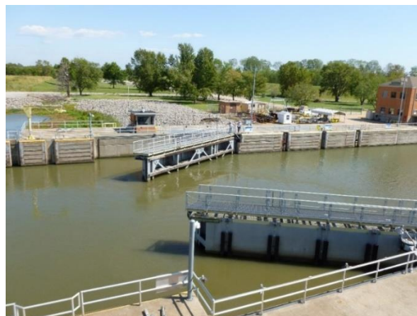
Newt Graham Lock and Dam No. 18, Fort Gibson, Oklahoma
