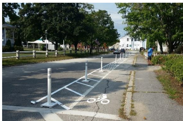
Demonstration project in Troy, New Hampshire
