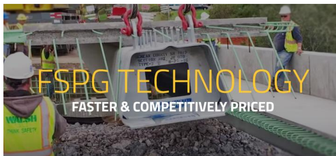
FSPGS with shorter length (less than 60 feet) was used in several bridges in 2016 and 2017 for replacing substandard bridges in Pennsylvania, as part of the State's major bridge replacement program.
