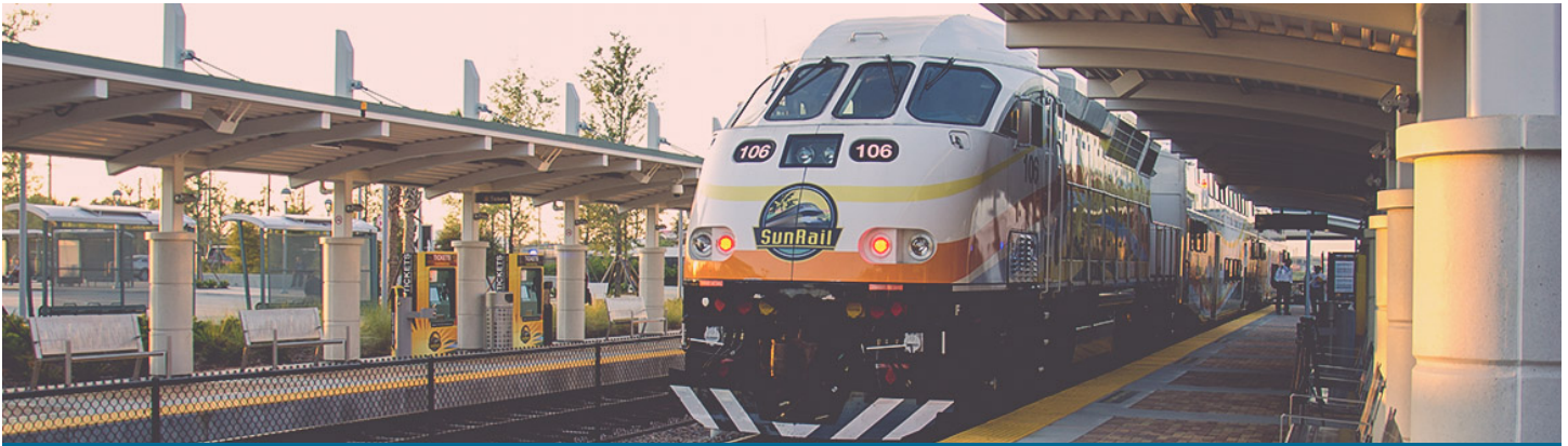
Florida's SunRail Commuter Rail began service in 2014.
