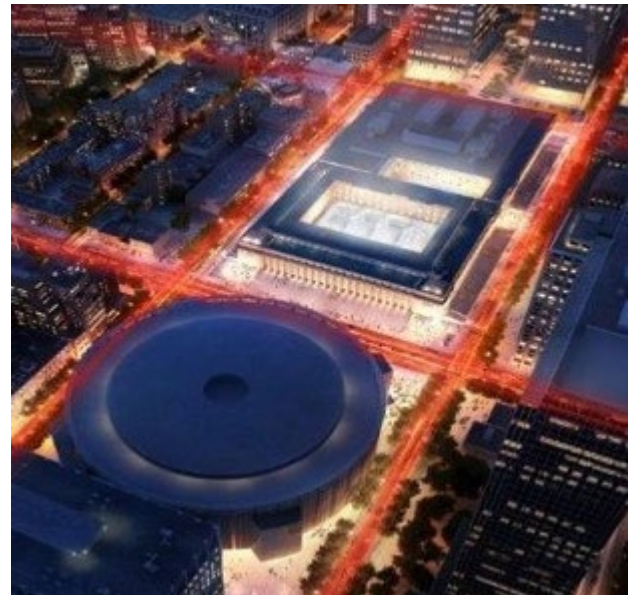
Moynihan Train Hall, the bright rectangle in the image above, will expand the capacity of the existing Penn Station, located below Madison Square Garden, the circular building in the image above.
