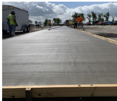
Construction of the Full-Scale, Jointless UTW-ECC Overlay
