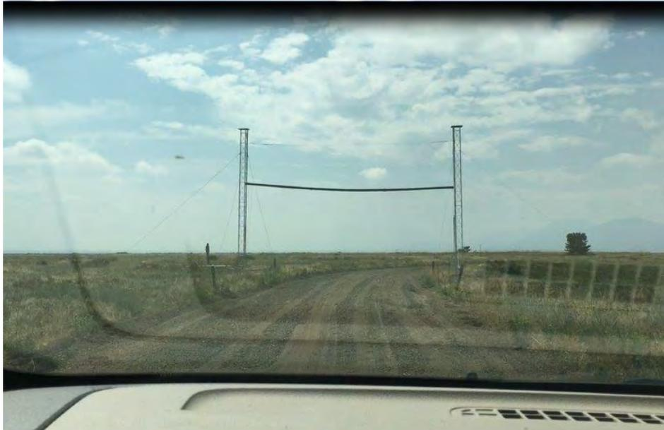
Figure 5-18. Rohn Model 25G towers with PVC RSU mounting pole
