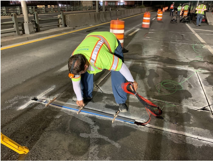
Installation of WIM System on Brooklyn-Queens Expressway
