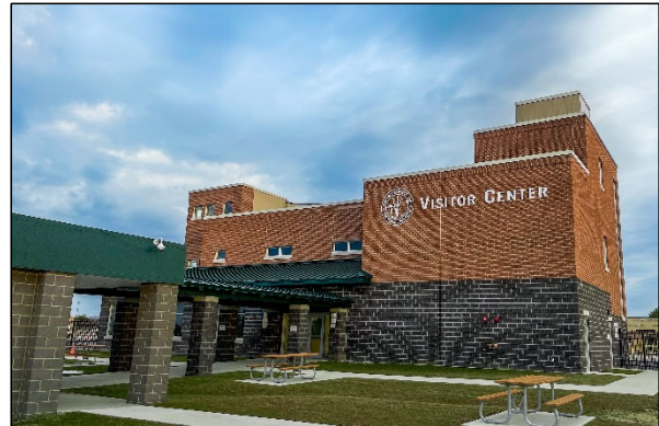
GLS's Seaway Visitor Center at Eisenhower Lock was completed in early FY 2024 and opened to the public in May 2024.
