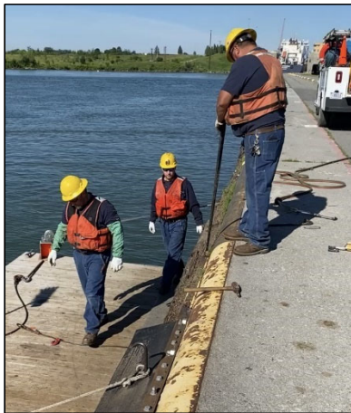
GLS work crews perform fendering replacement along the lower guidewall at Eisenhower Lock.
