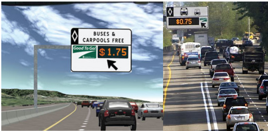
Figure 2: A rendering of HOT facility by WSDOT; A HOT lanes facility on SR 167 in Washington (4)
